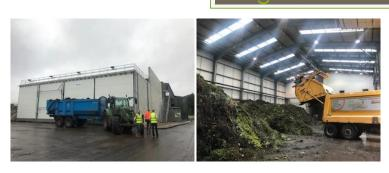
The application site area is approximately 1.2 hectares. The application proposes to develop an organic waste in vessel composting (IVC) facility to manage up to 75,000 tonnes per annum of compostable municipal green and food waste. This would involve a mixture of invessel composting (IVC) within a purpose built building, and external aerated maturation using a system of forced aeration static windrows.
